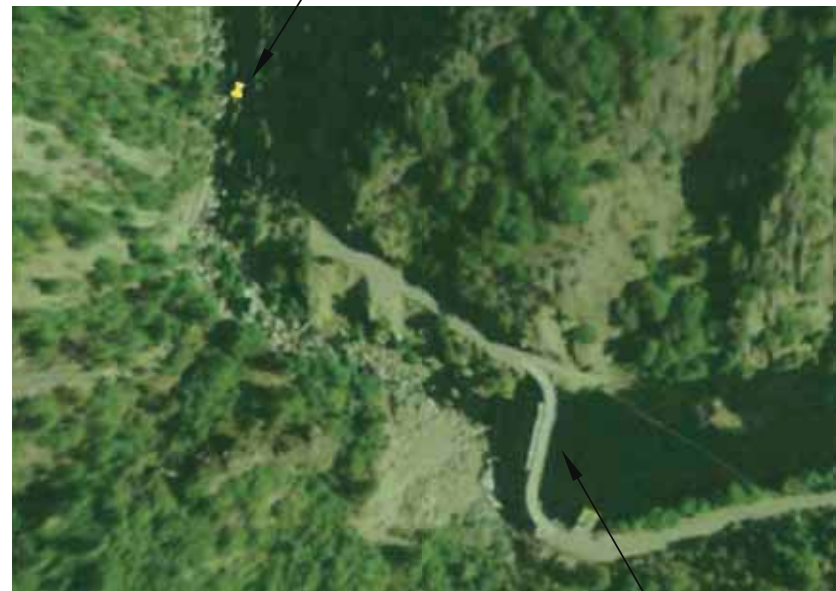
INTERBAY DAM & DOWNSTREAM VICINITY
