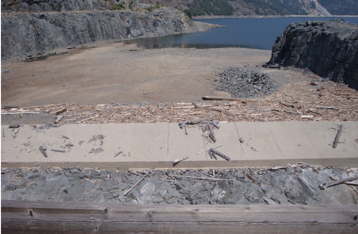
Figure 2-3 - Hell Hole Spillway Approach Channel
