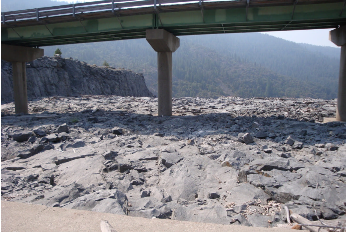
Figure 2-5 Spillway Discharge Channel showing Invert Roughness @ Bridge Crossing
