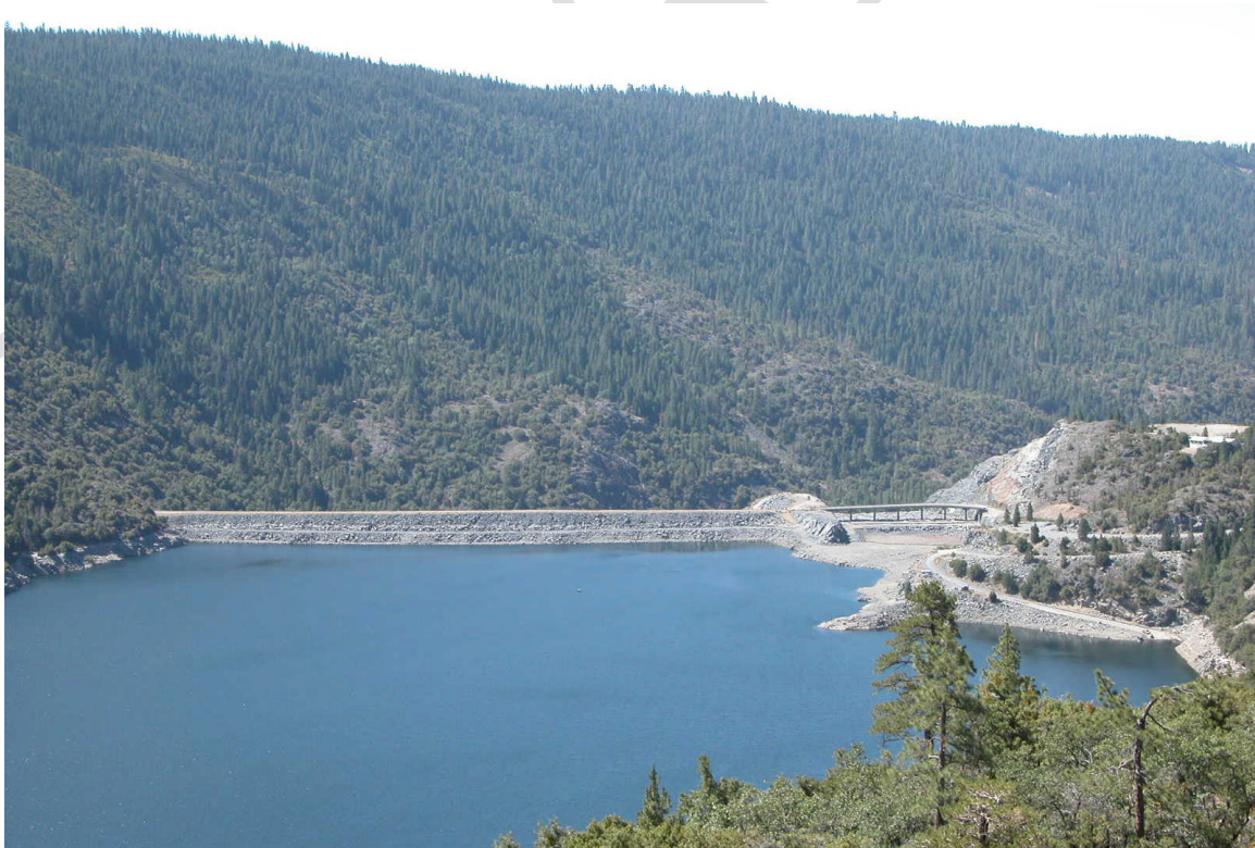
Figure 2-2 - View from upstream of Hell Hole Dam and Spillway
