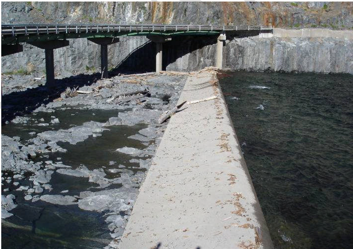
Figure 2-4 - Hell Hole Spillway Weir
