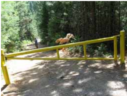
NFLCCRSNRPA02 – North Fork Long Canyon Crossing Removable Section North Road and Parking Area at Road Mile 0.007
