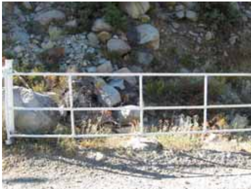
FMPR48 – French Meadows Powerhouse Road at Road Mile 1.212
