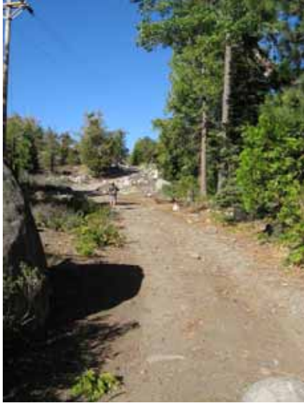
FR14N09A01 – Forest Road 14N09A at Road Mile 0.000
