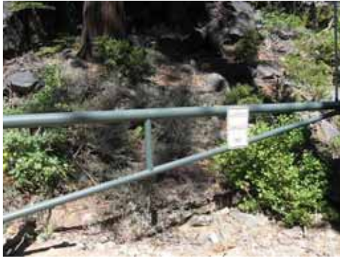
HHMFTGR05 – Hell Hole–Middle Fork Tunnel Gatehouse Road at Road Mile 0.030
