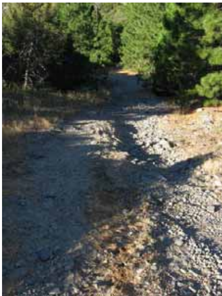
HHSDCR04 – Hell Hole Dam Spillway Discharge Channel Road at Road Mile 0.055
