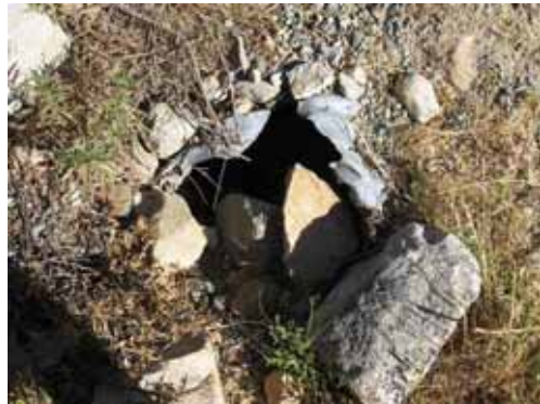
FMPR52 – French Meadows Powerhouse Road at Road Mile 1.275
