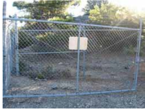
DFR06 – Dormitory Facility Road at Road Mile 0.127
