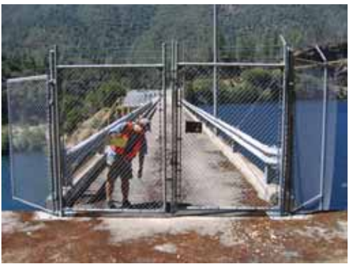
RADRAAP02 – Ralston Afterbay Dam Road and Afterbay Access Point at Road Mile 0.119
