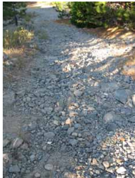
HHSDCR05 – Hell Hole Dam Spillway Discharge Channel Road at Road Mile 0.087
