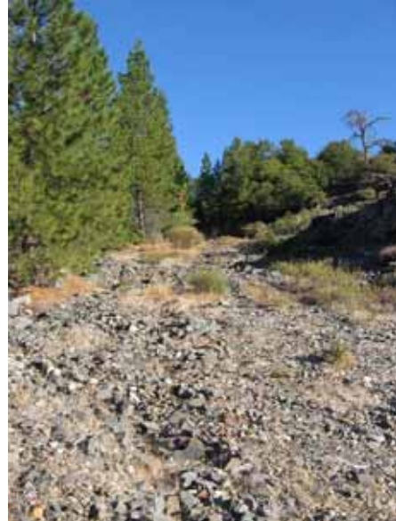
HHSDCR09 – Hell Hole Dam Spillway Discharge Channel Road at Road Mile 0.182
