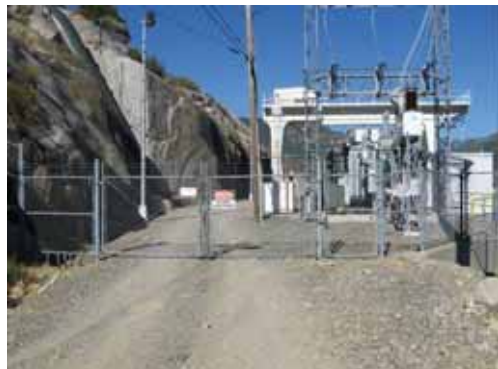
FMPR54 – French Meadows Powerhouse Road at Road Mile 1.280
