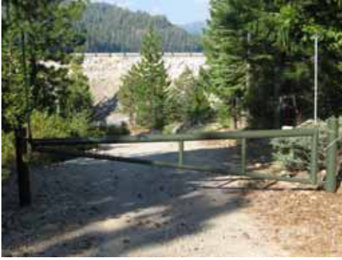
FMDOWLWR02 – French Meadows Dam Outlet Works and Leakage Weirs Road at Road Mile 0.007
