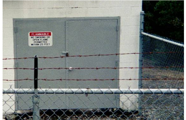
Photo 30. Sign is located on the door on east side of Ralston Afterbay Dam Generator Building.
