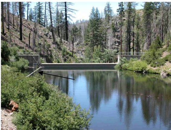
DDD1 – Log boom across spillway at Duncan Creek Diversion Pool.
