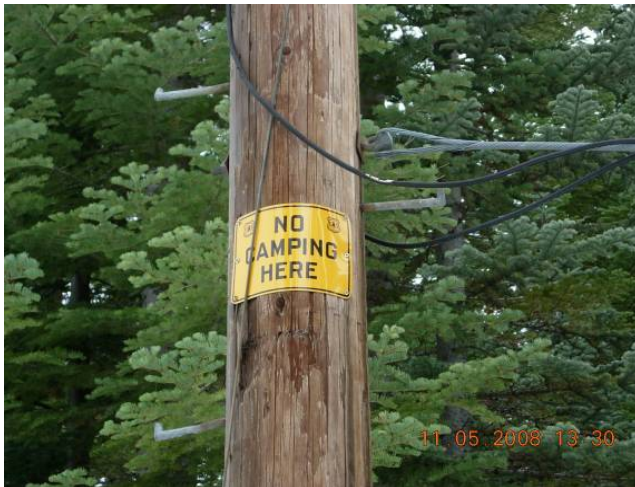
Photo 13. Sign is located on the radio communications pole near the Radio Communications Tower near French Meadows – Hell Hole Tunnel Powerhouse.
