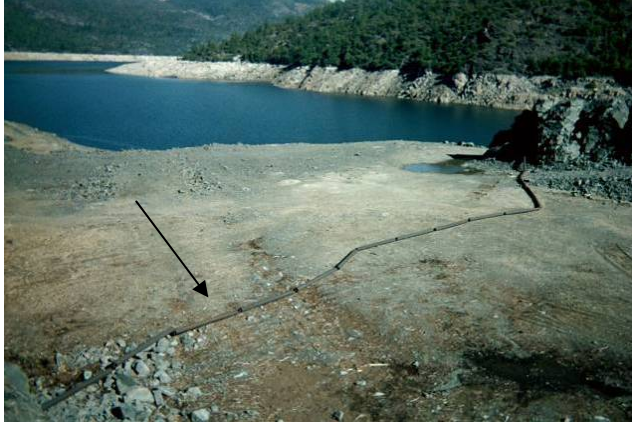
HHD1 – Log boom across spillway at Hell Hole Reservoir.
