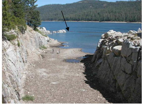
FMD1 – Log boom across spillway at French Meadows Reservoir.
