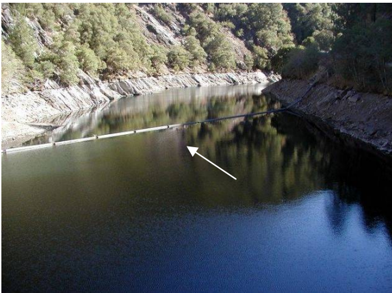
MFID1 – Log boom across spillway at Middle Fork Interbay.
