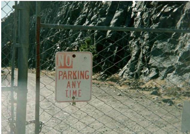
Photo 3. Sign is located on gate on Hell Hole Dam and Powerhouse Road.
