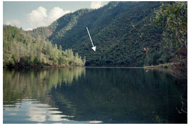
RAD1 – Log boom across spillway at Ralston Afterbay
