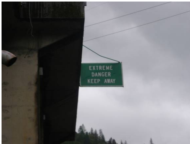
Photo 27. Sign is located on the stream side of Ralston Powerhouse.
