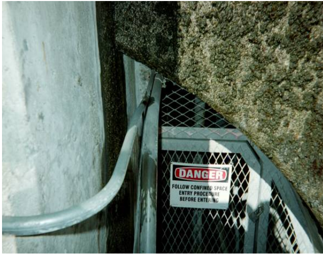
Photo 5. Sign is on the gate leading into tunnel at the back of Hell Hole Powerhouse.
