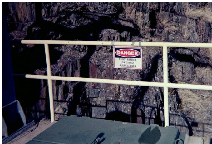
Photo 31. Sign is located on the railing around Ralston – Oxbow Tunnel Intake.
