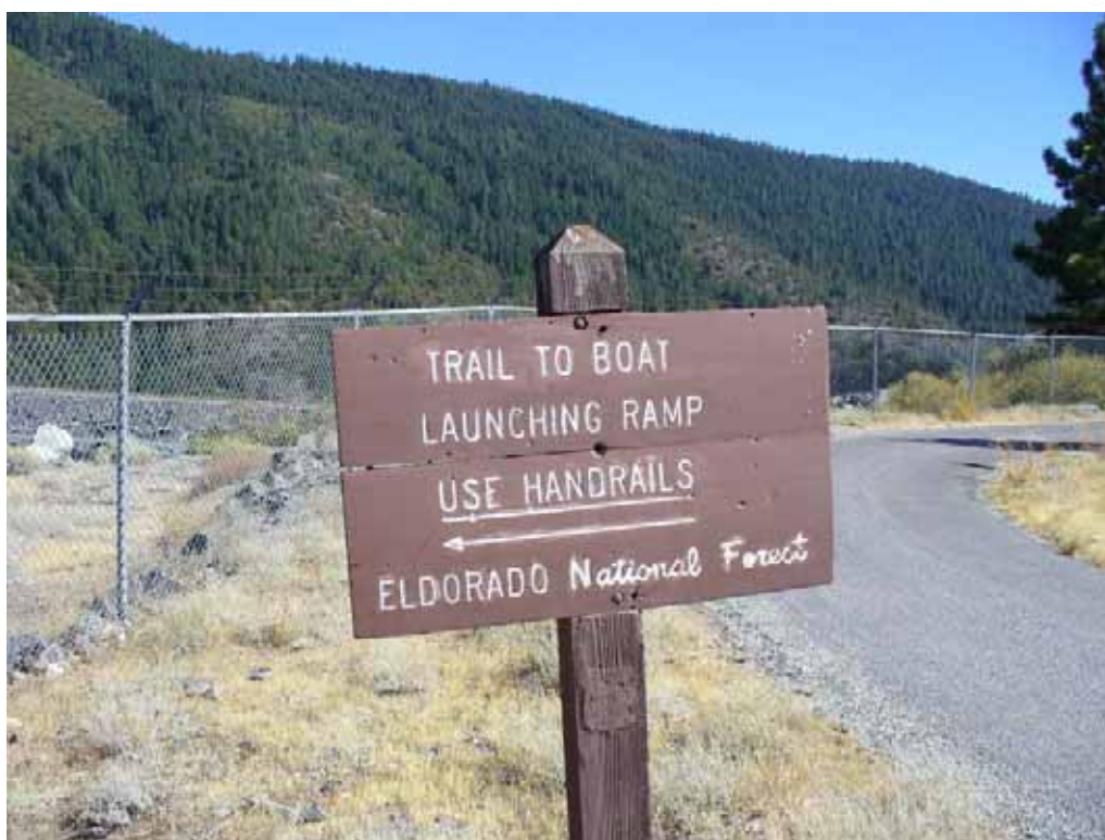
Photo H-2-30. Directional sign at entrance to trail/stairway to Hell Hole Boat Ramp. Sign is constructed of painted wood on wood post. Sign is in fair condition due to split boards and faded lettering. (8/4/08)
