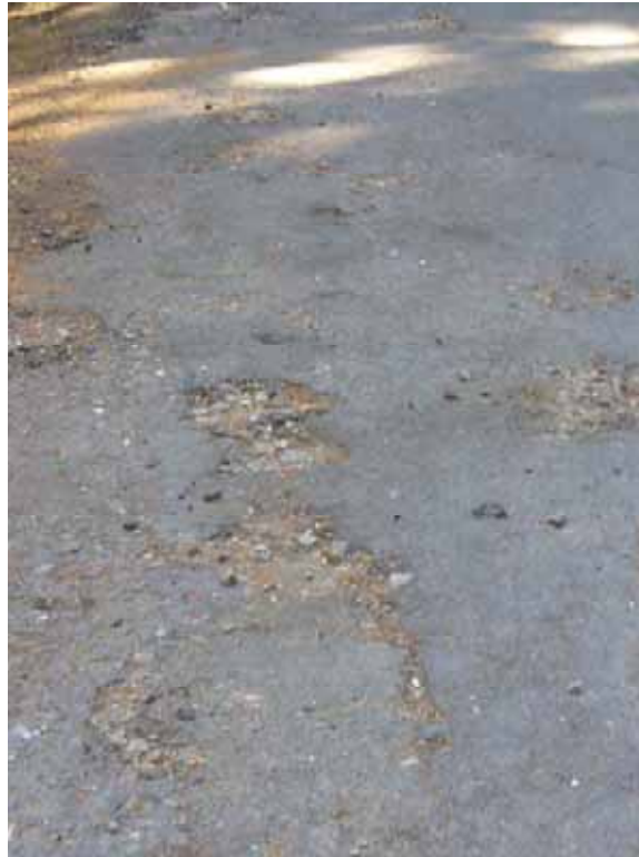
Photo E-2-7. Poor condition pavement at edge of Hell Hole Campground Parking Area. (8/21/08)
