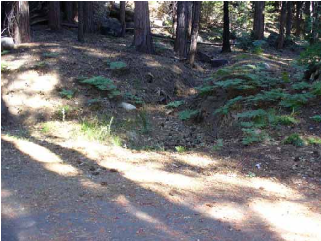
Photo E-2-10. Drainage into parking area. (8/21/08)
