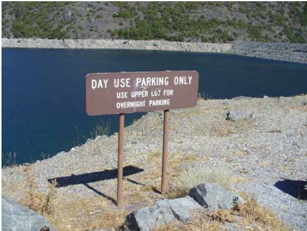
Photo H-2-15. Regulatory sign in lower parking lot. Constructed of painted MDO on steel posts. Good condition. (8/4/08)
