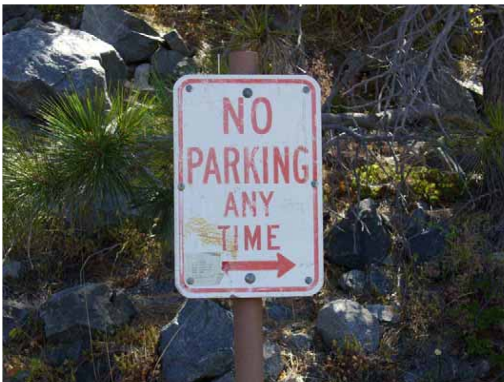
Photo H-2-2. Example of “no parking” sign located along Hell Hole Boat Ramp. Condition is “fair” due to faded lettering. (8/4/08)
