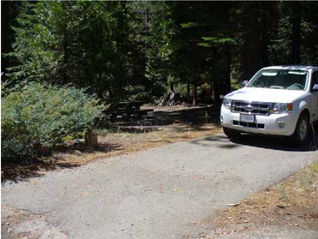
Photo D-2-8. Example campsite parking spur (Site 1). This spur is a “trailer spur”, 40’ long x 10’ wide. (8/21/08)
