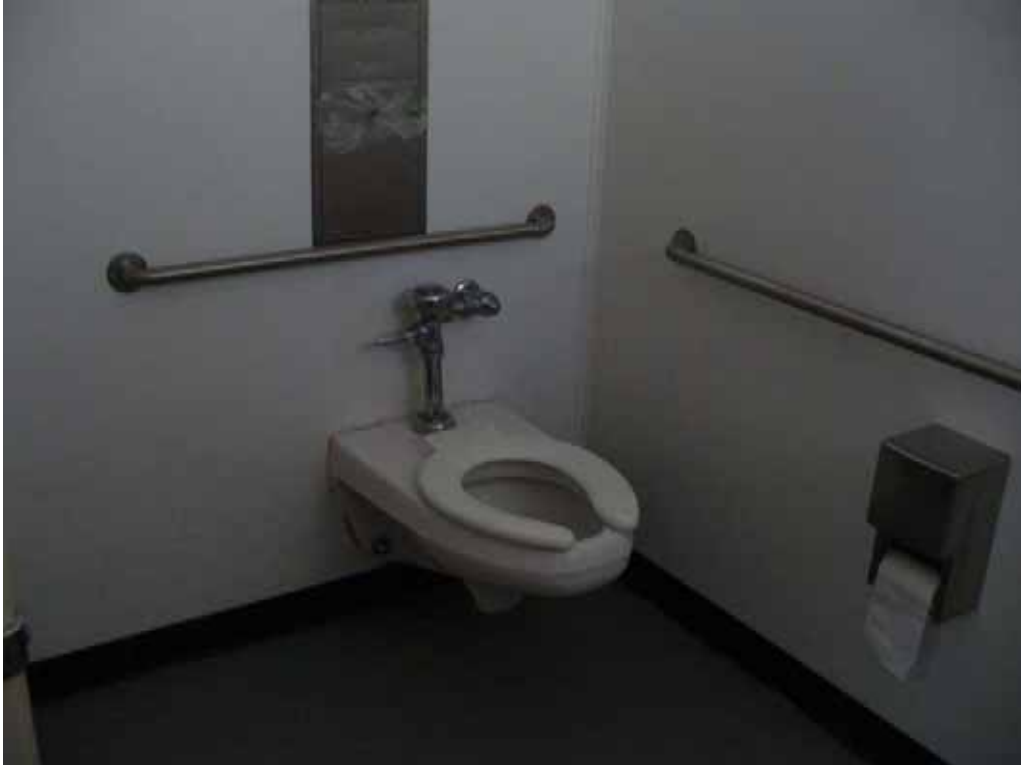
Photo K-2-18. Inside of wood bathroom structure converted to meet accessibility standards. (9/04/08)
