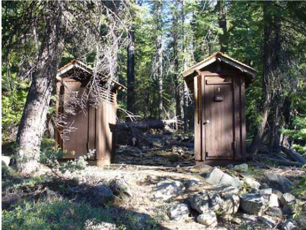
Photo L-2-14. Pit toilets in campground. No accessible. (7/24/08)
