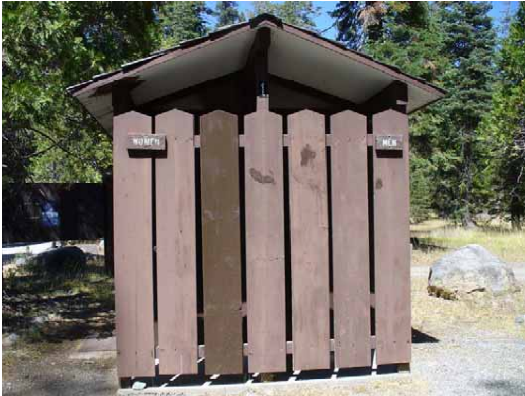
Photo I-2-13. Double-unit, vault toilet building (No. 1). (9/04/08)
