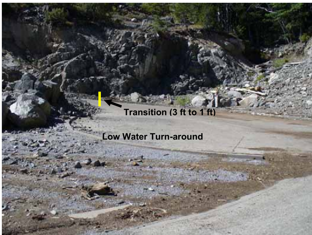
Photo H-2-4. Low water turn-around area in apex of ramp. Note that masonry retaining wall transitions from 3-foot high to 1-foot high. (8/4/08)
