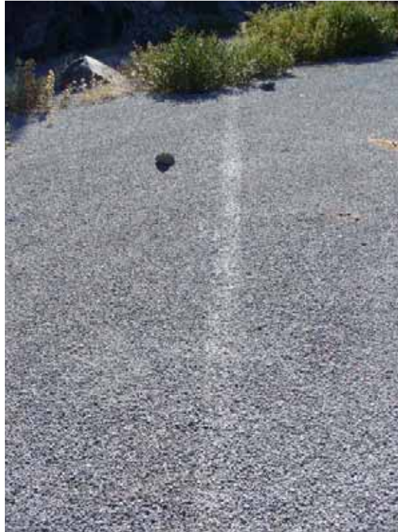
Photo H-2-26. Example of faded parking stall striping on asphalt with chip seal. (8/4/08)
