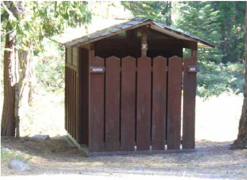
Photo K-2-10. Wood bathroom structure No. 2. This is a double unit vault toilet in fair condition. Not accessible. (9/04/08)
