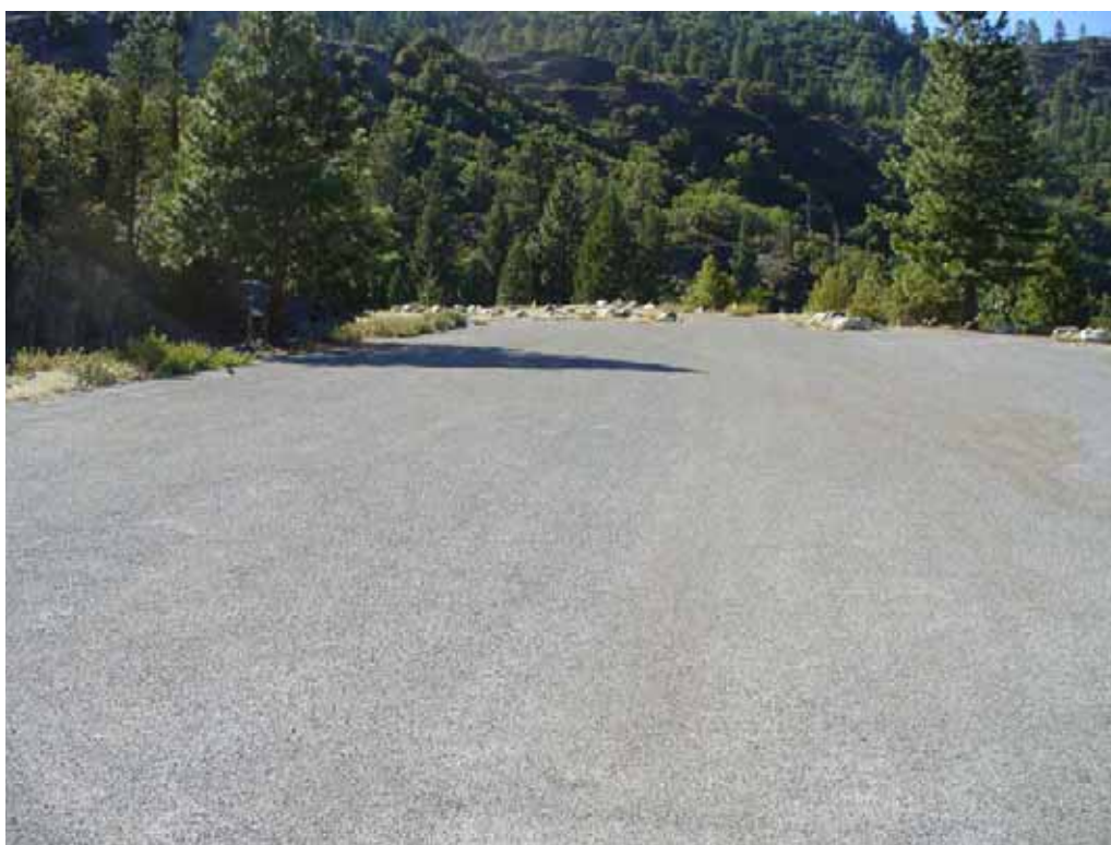
Photo H-2-22. Hell Hole Boat Ramp General Parking Area (northern portion). Surface is asphalt with chip seal in good condition. (8/4/08)
