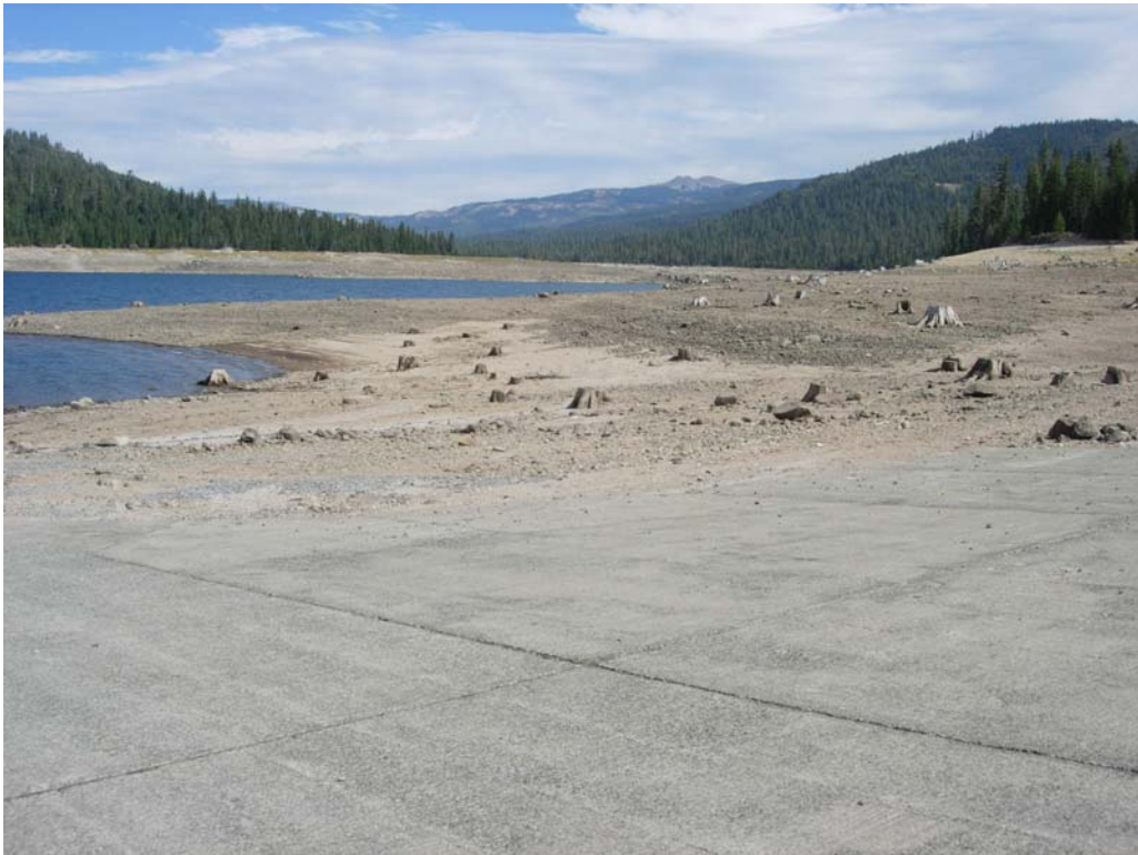
Photo G-6. View of reservoir from French Meadows Boat Ramp on September 24, 2008 (WSE = 5,198 ft).
