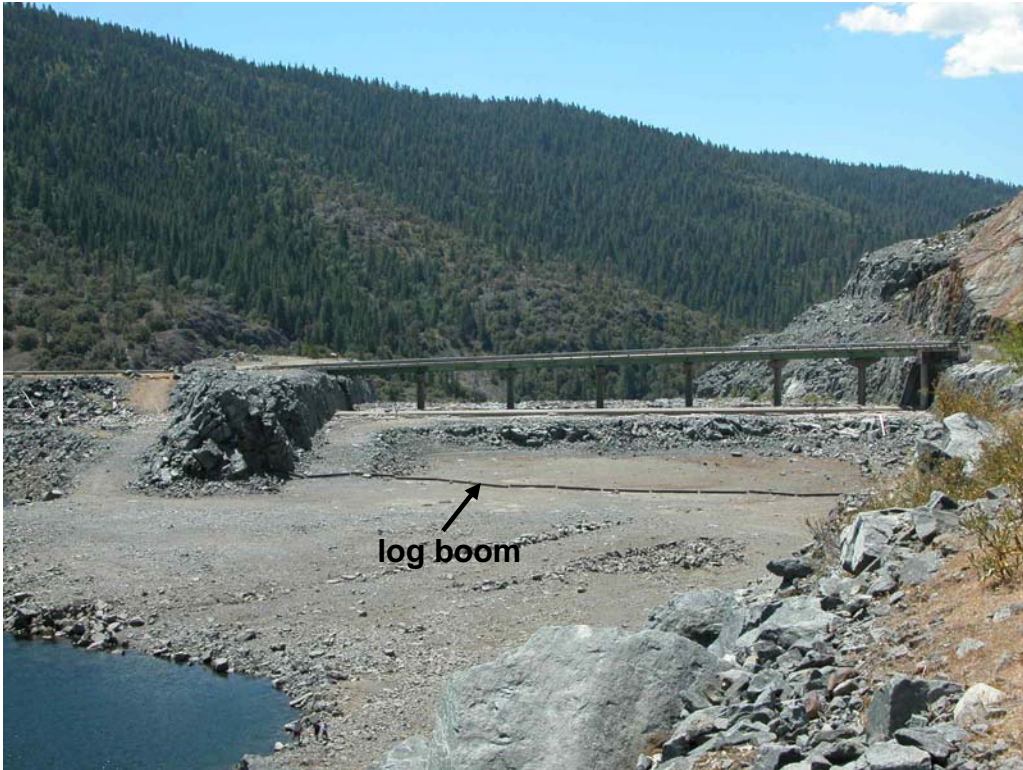
Photo E-1. View of log boom near spillway at Hell Hole Reservoir.
