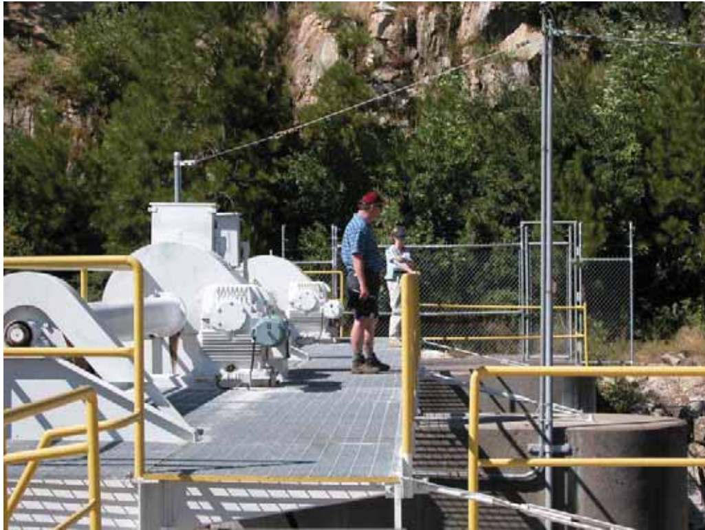
Photo J-2. View of public safety fence and railing surrounding French Meadows Spillway Gates area.
