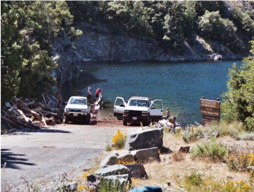
Photo B-1. Top of Hell Hole Boat Ramp as viewed from near Hell Hole Boat Ramp Parking Area. Reservoir is almost at maximum operating WSE of 4,630 feet. Note transition from top of concrete ramp to asphalt pavement (date of photo unknown, WSE ~ 4,628).
