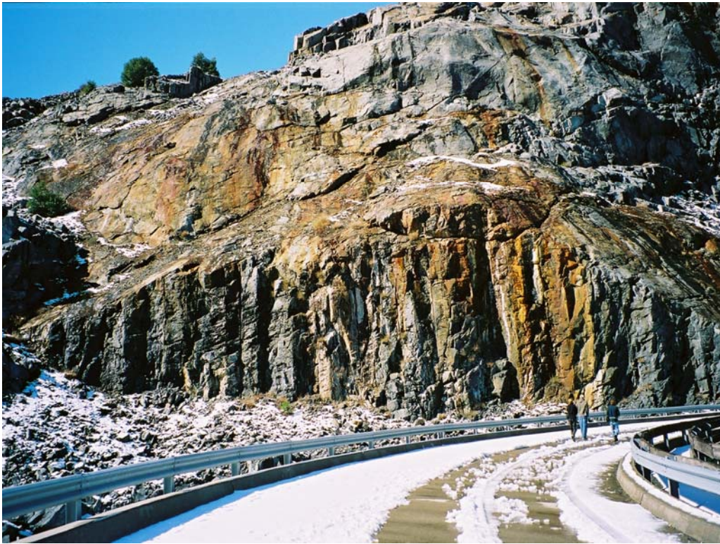
Photo E-4. View of guard rails along top of Hell Hole Dam.
