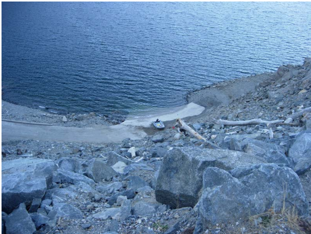
Photo B-6. Bottom End of Boat Ramp (October 13, 2008, WSE = 4,536 ft)
