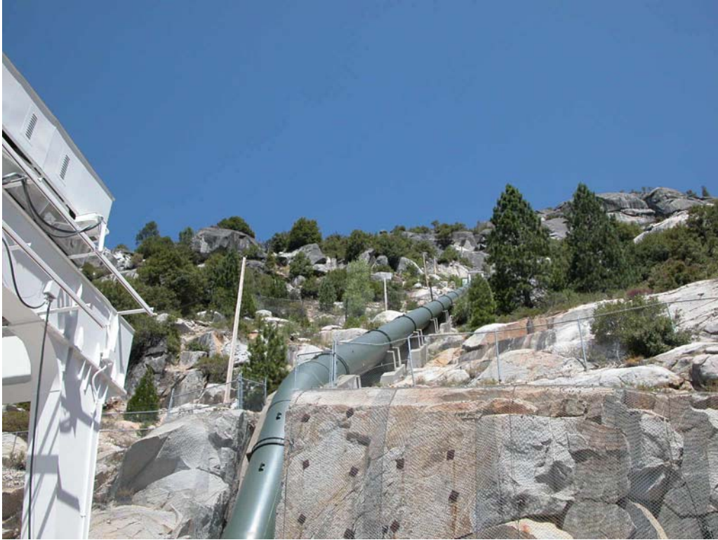
Photo E-3. View of slope fence adjacent to French Meadows Powerhouse.
