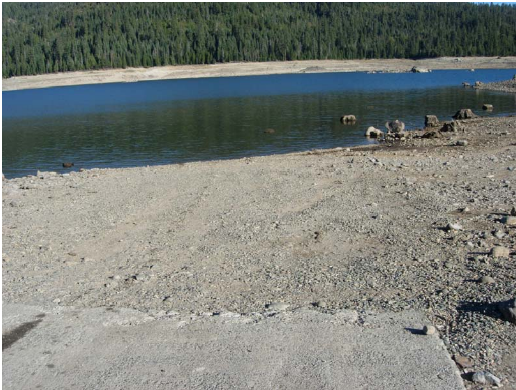
Photo G-8. French Meadows Boat Ramp on October 14, 2008 (WSE = 5,193 ft). Note that boat launching is still possible after the WSE declines below the end of the concrete ramp due to the compacted substrate and shallow slope of shoreline.
