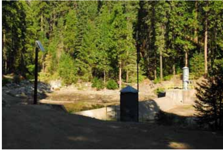
North Fork Long Canyon Creek Diversion Pool
