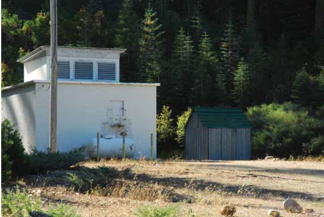
French Meadows - Hell Hole Tunnel Inlet Gatehouse
