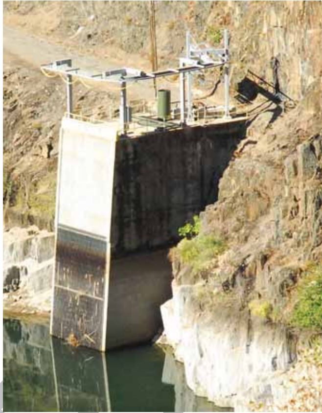
Ralston-Oxbow Tunnel Inlet Structure
