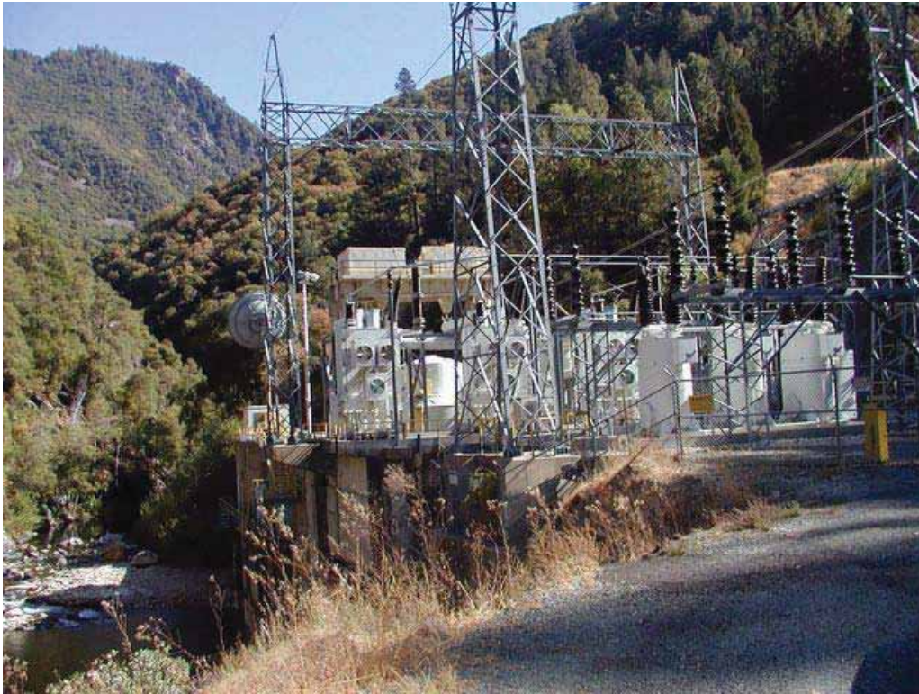
Middle Fork Powerhouse
