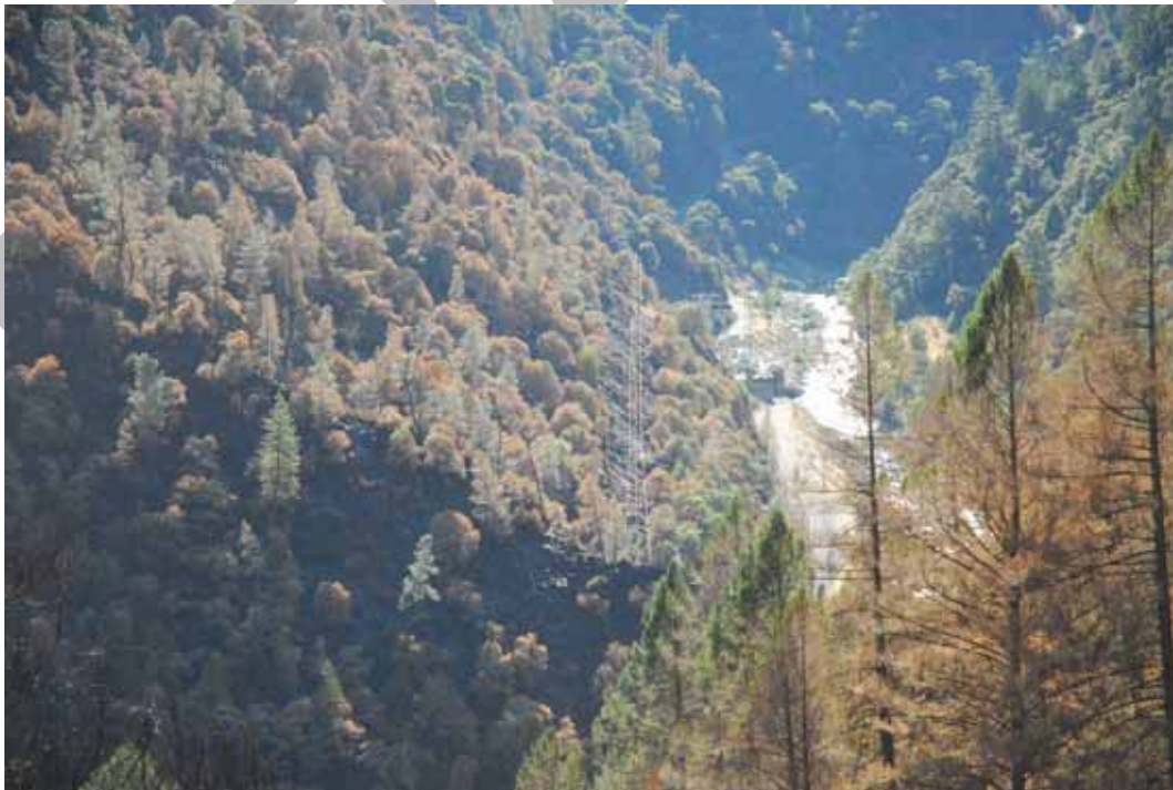
Ralston Powerhouse with Low Water Level
