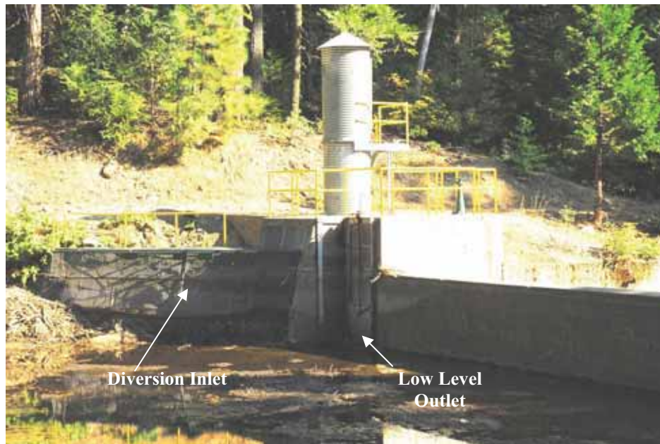
North Fork Long Canyon Diversion – Downstream Side
