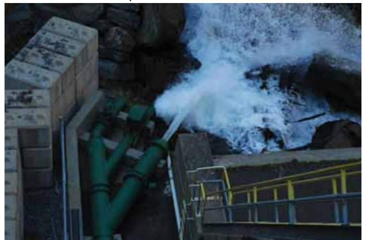
Instream Flow Pipes
