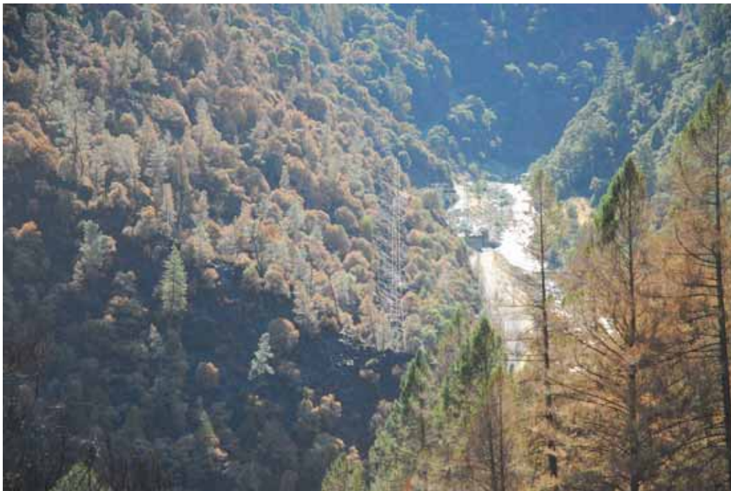
Ralston Powerhouse with Low Water Level
