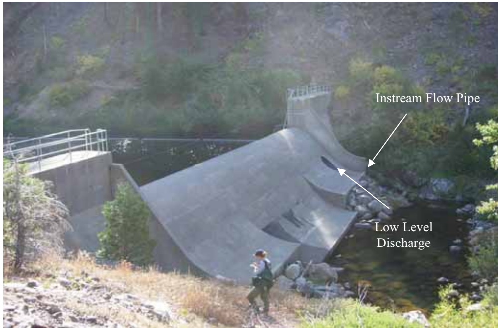
Duncan Creek Diversion Dam – Downstream Side
