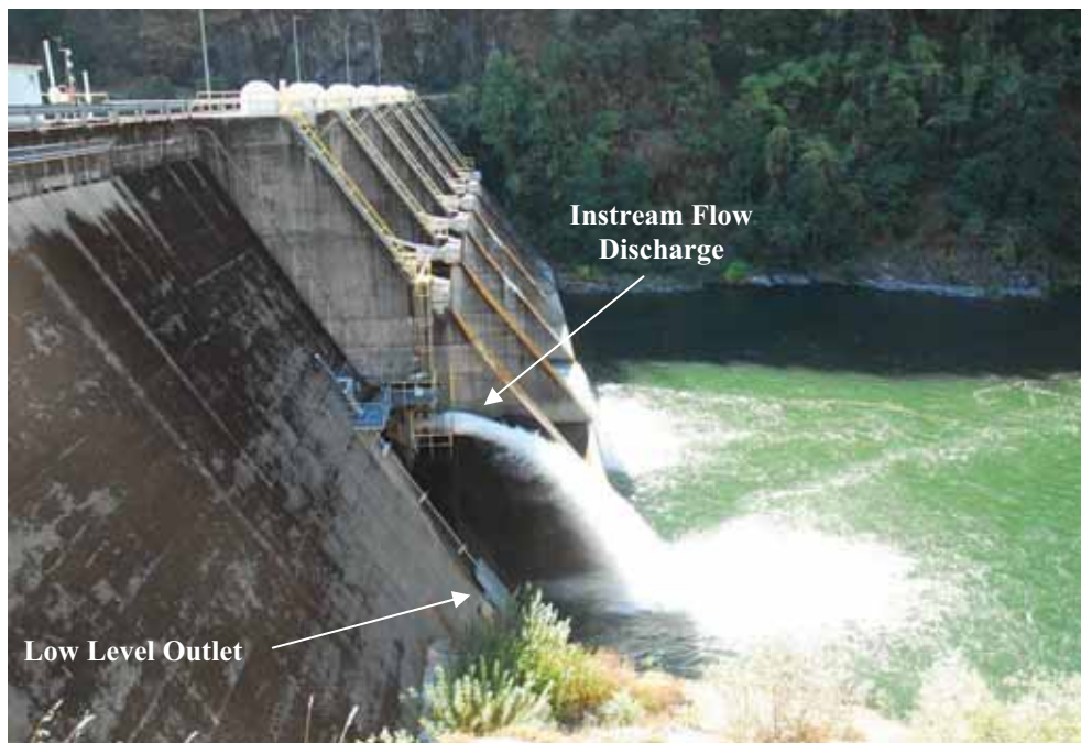
Ralston Afterbay Dam – Downstream
