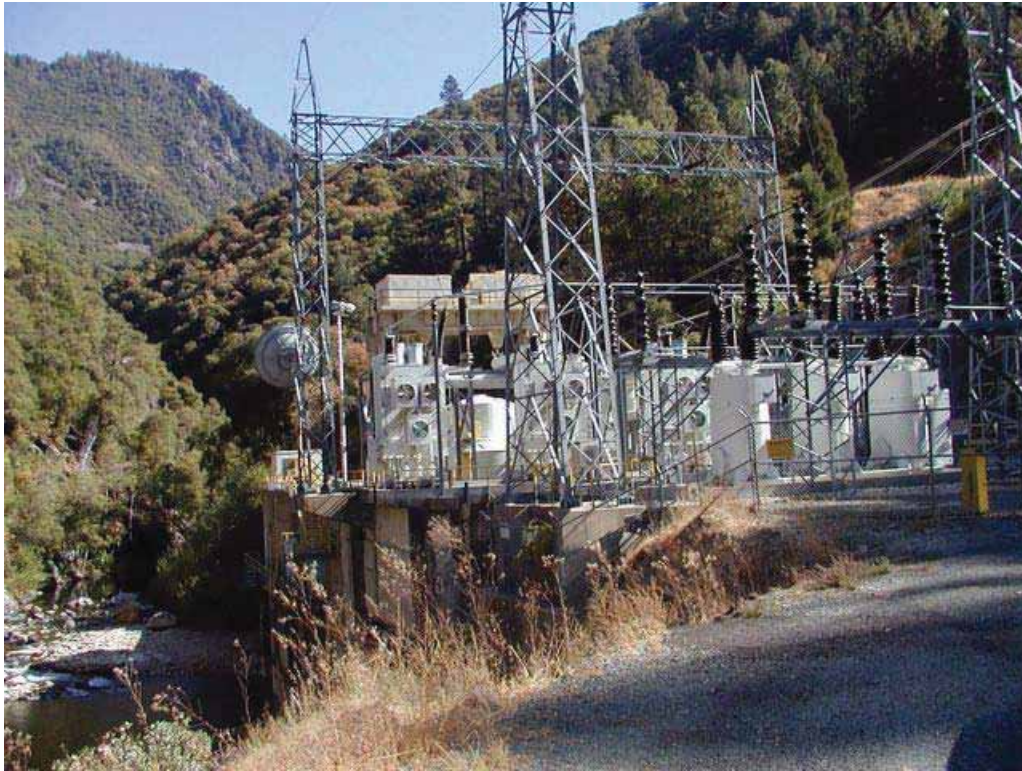
Middle Fork Powerhouse
