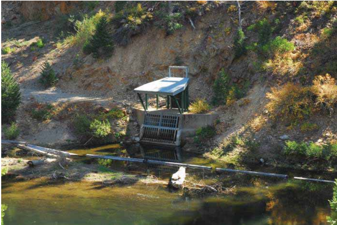
Duncan Creek - Middle Fork Tunnel Intake
