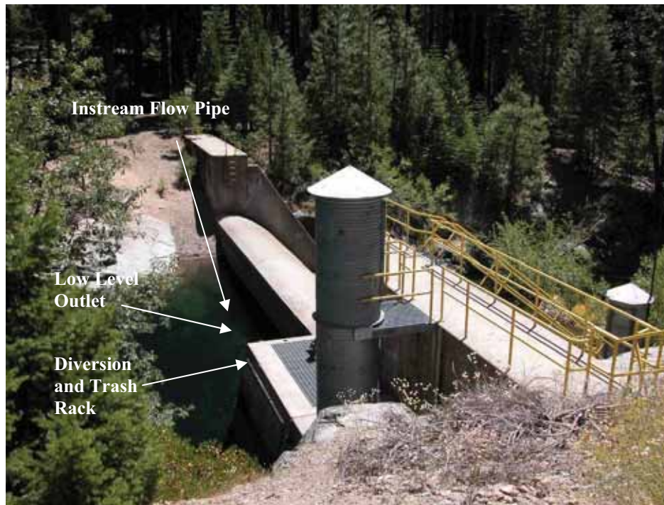
South Fork Long Canyon Diversion Dam
