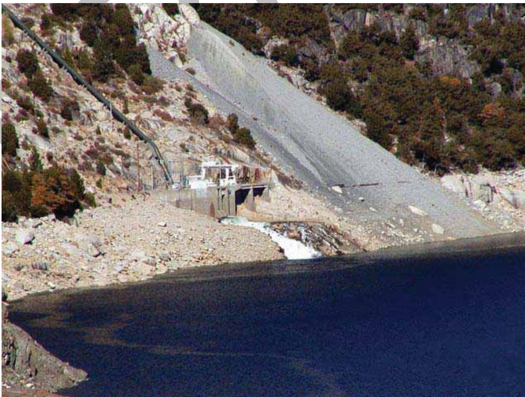
French Meadows Powerhouse
