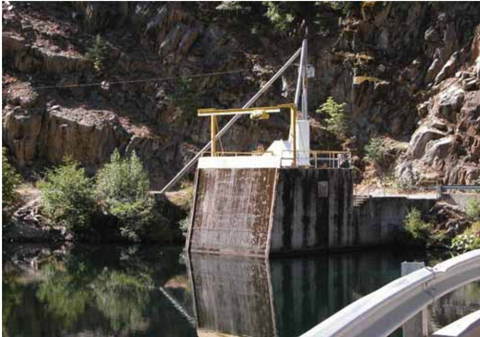
Middle Fork – Ralston Tunnel Inlet Structure
