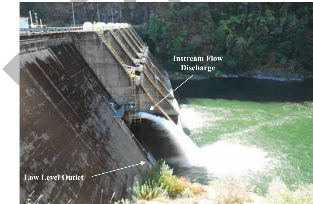
Ralston Afterbay Dam - Downstream
