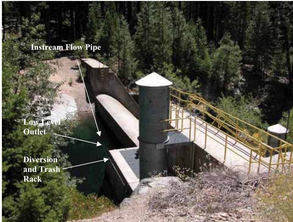
South Fork Long Canyon Diversion Dam
