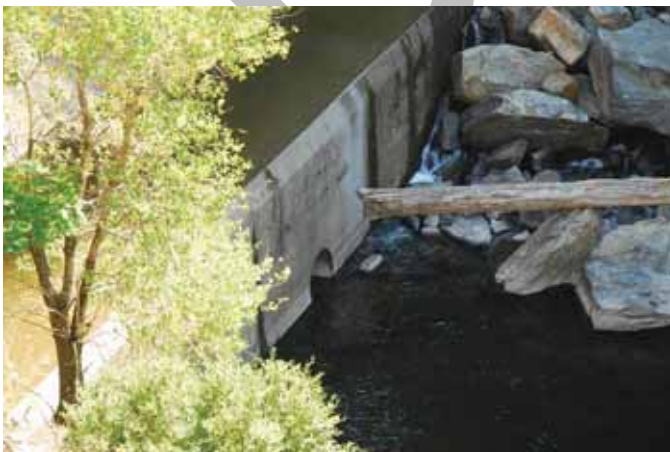
Interbay Dam Low Level Discharge
