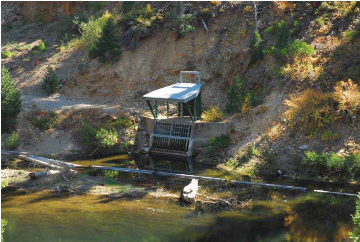
Duncan Creek – Middle Fork Tunnel Intake
