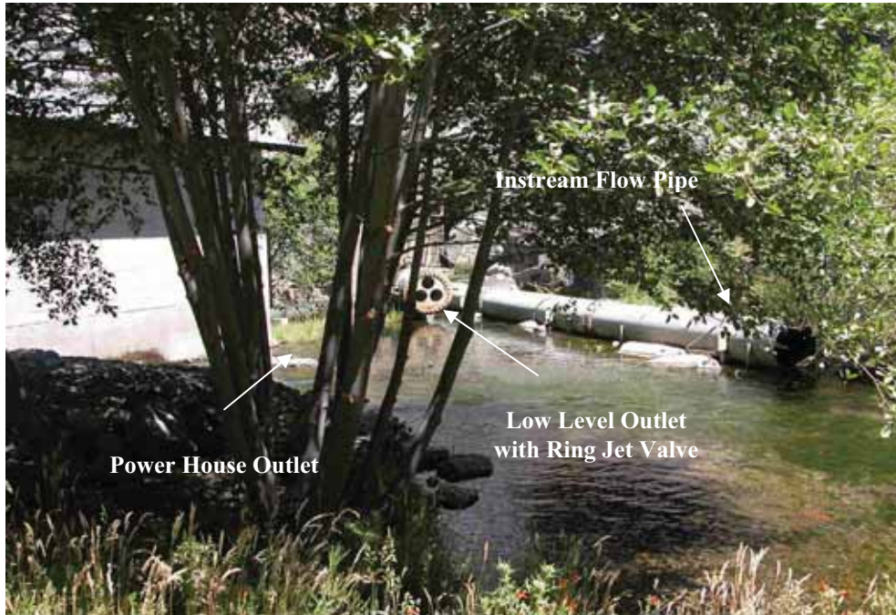
Dam Outlet Works
