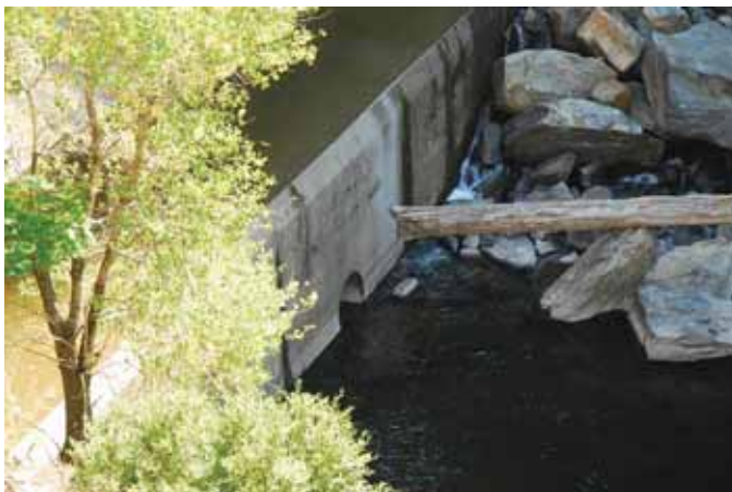
Interbay Dam Low Level Discharge
