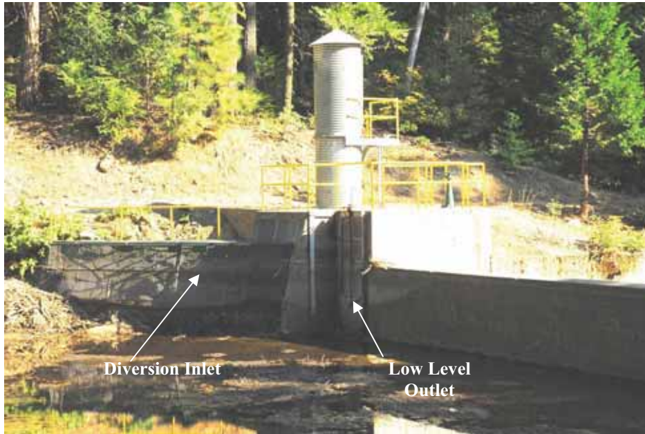
North Fork Long Canyon Diversion - Downstream Side
