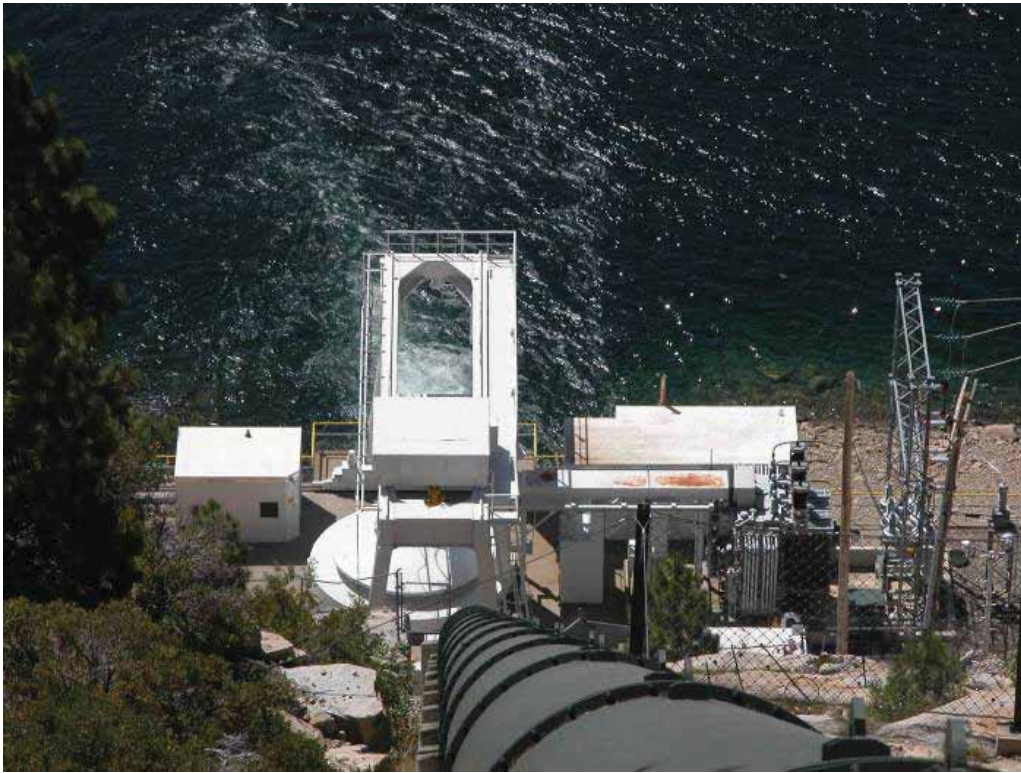
French Meadows Powerhouse
