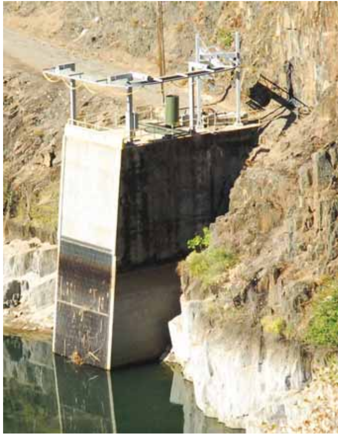
Ralston – Oxbow Tunnel Inlet Structure
