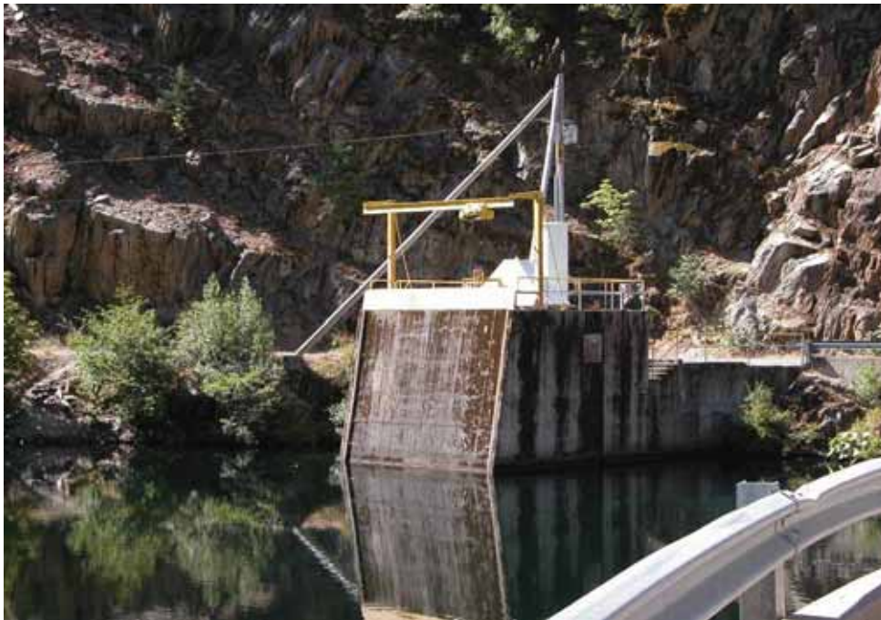
Middle Fork - Ralston Tunnel Inlet Structure
