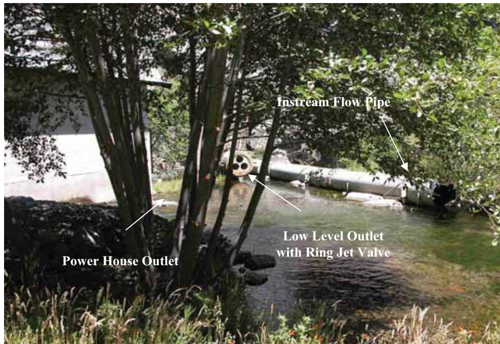
Dam Outlet Works
