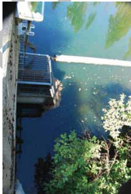
Inlet to Upstream Flow Pipe
