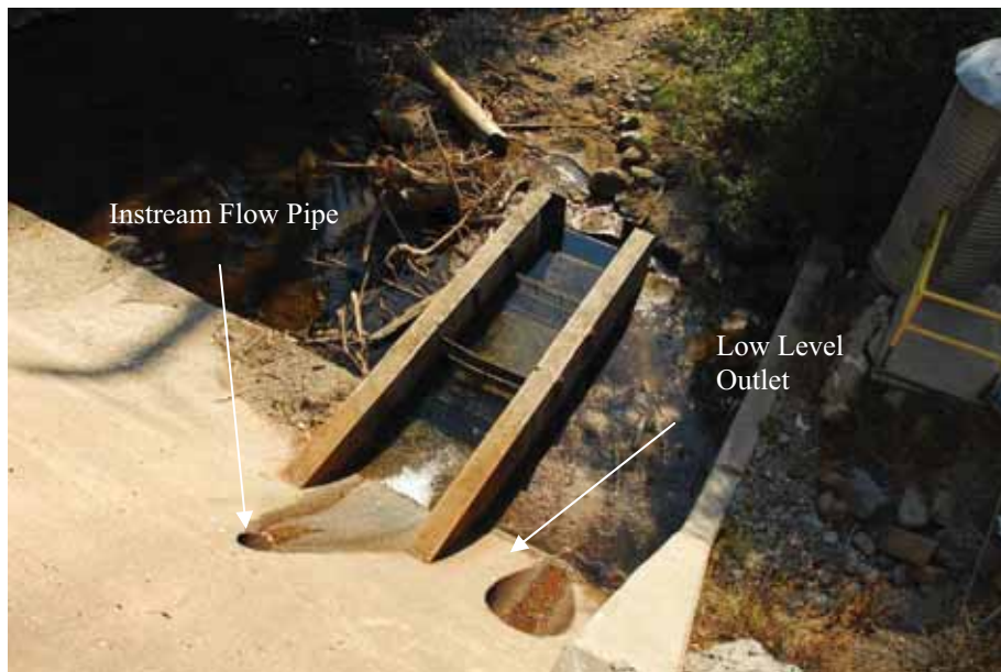
South Fork Long Canyon Diversion Dam – Downstream Side
