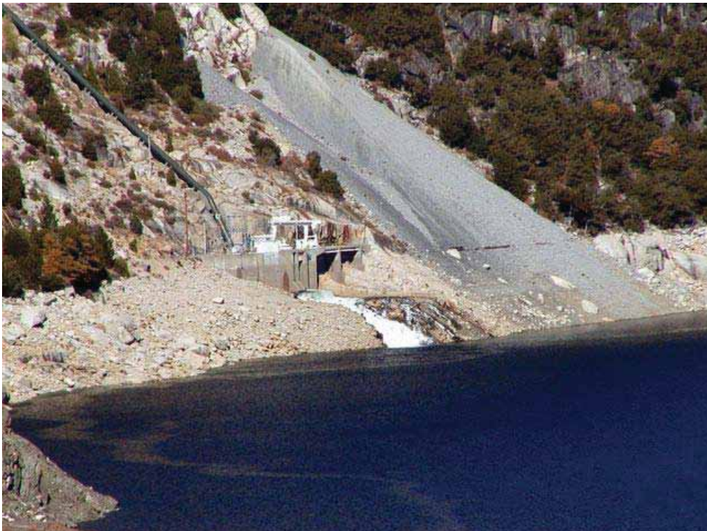
French Meadows Powerhouse
