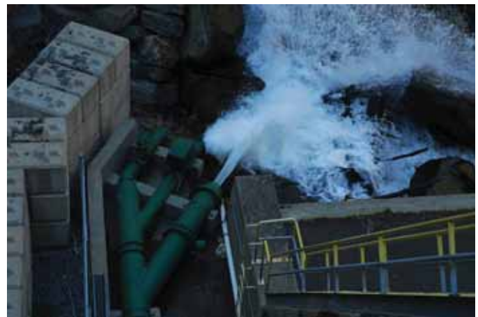
Instream Flow Pipes
