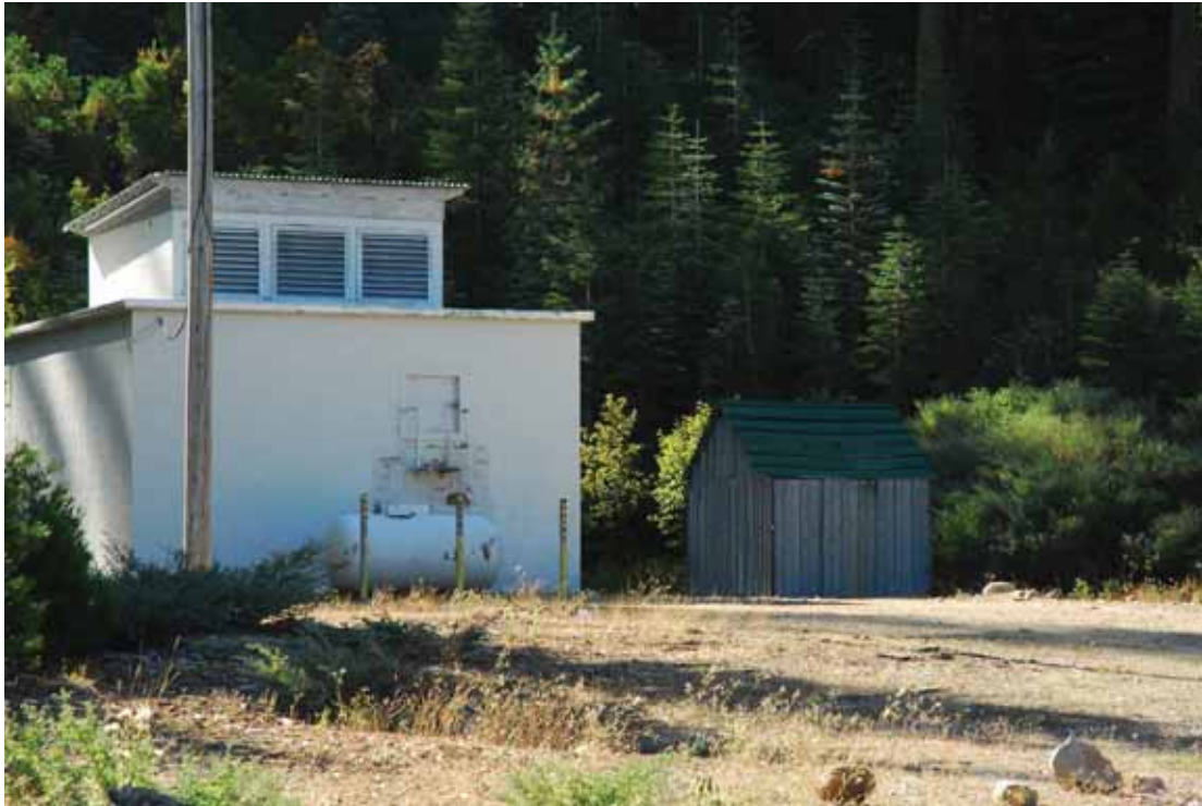
French Meadows - Hell Hole Tunnel Inlet Gatehouse
