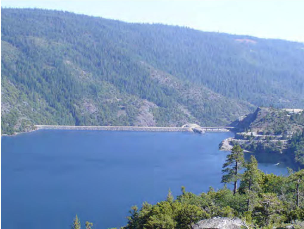
Figure 3.11-1. Existing dam and spillway with current maximum normal operating WSE (No-Action Alternative).
